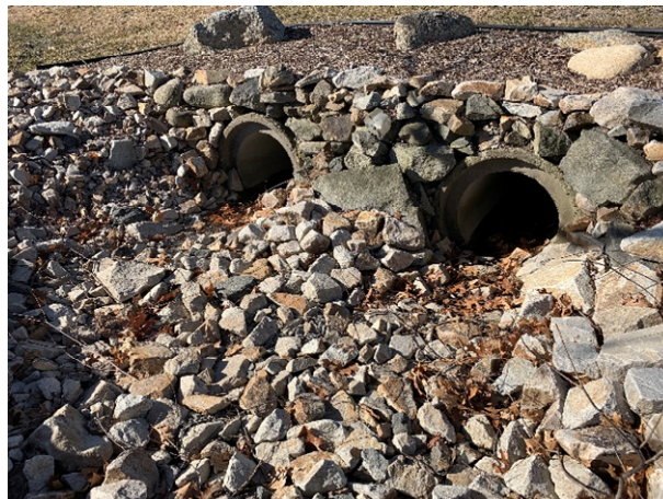
64 Gundalow - 2 (Drainage Course)
