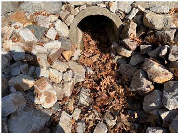
64 Gundalow - 1 (Drainage Course)
