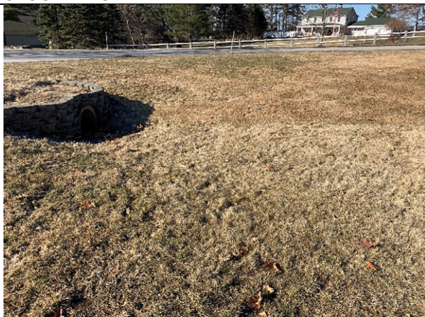
29 Gundalow - 1 (Drainage Area)
